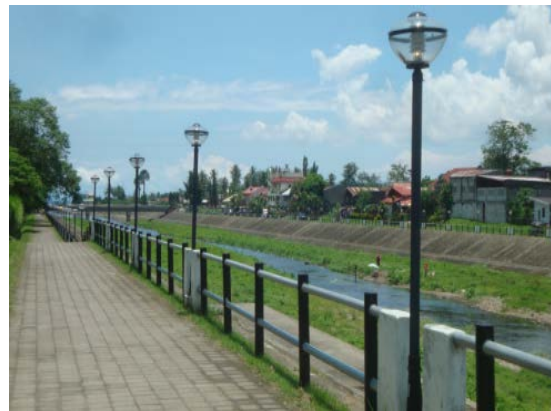
Ormoc Flood Mitigation Project
